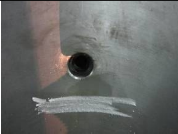
Water seal testing (No leakage)
