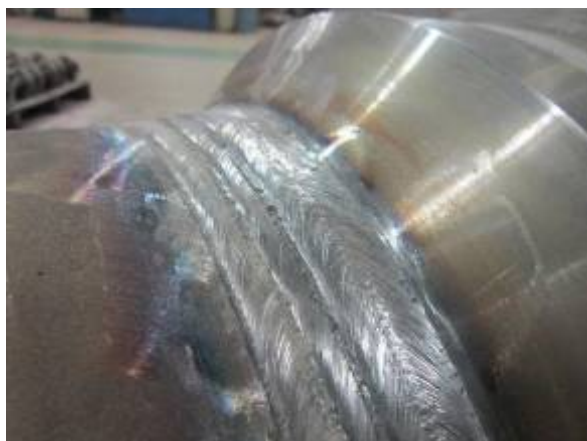
Weld seam check
