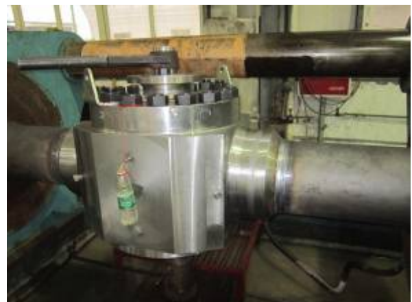
DBB air seal testing (No leakage)
